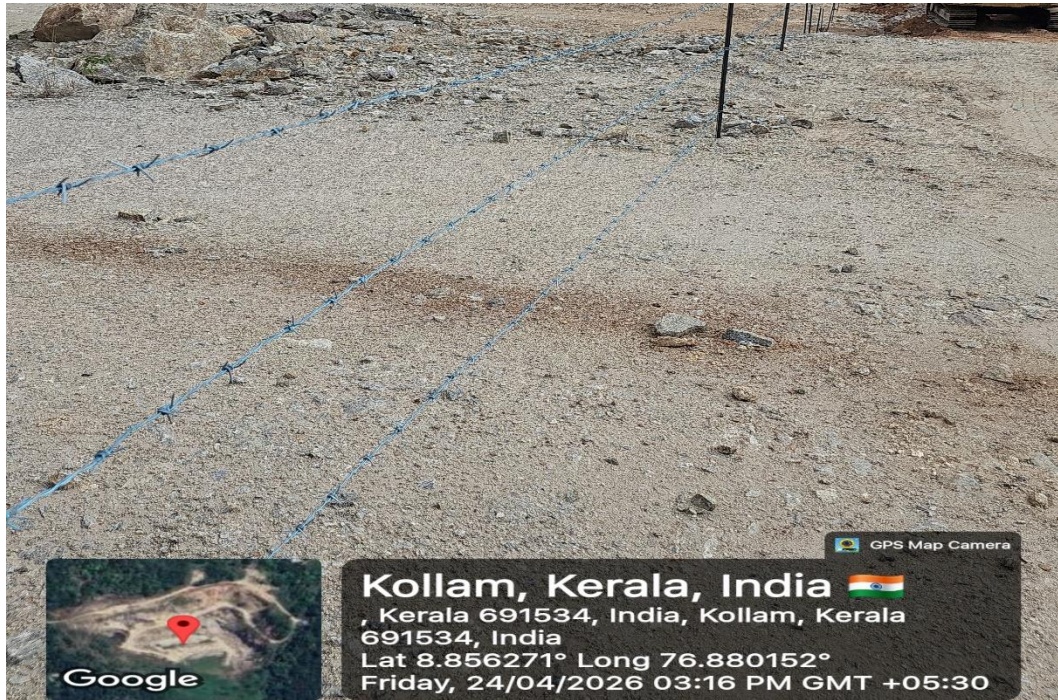
Figure 5 : Photograph of fencing provided
