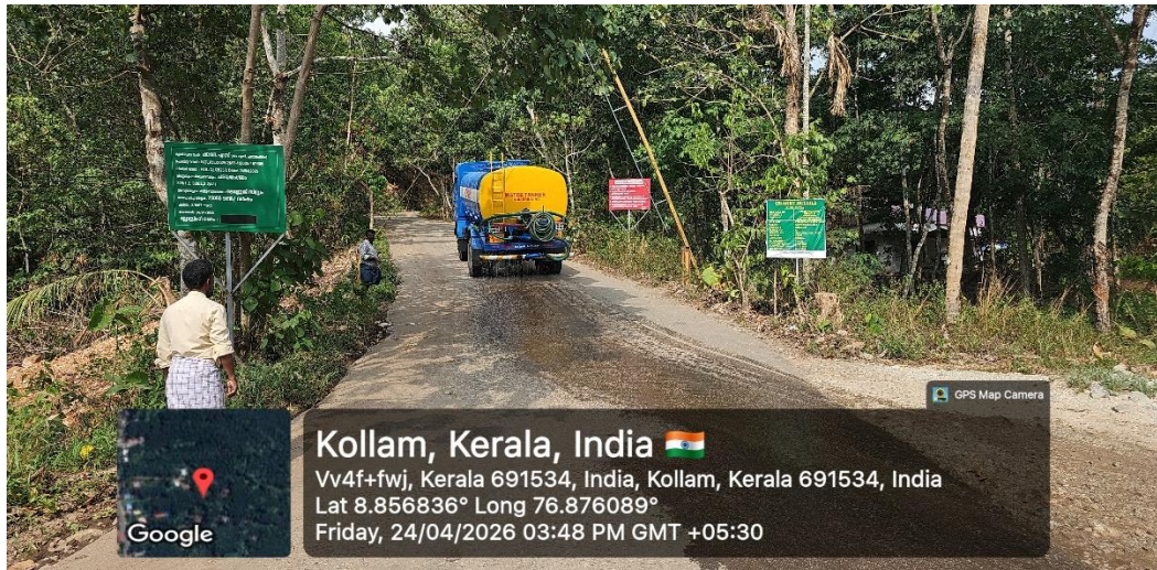
Figure 14 : Photograph of water spraying on haul roads
