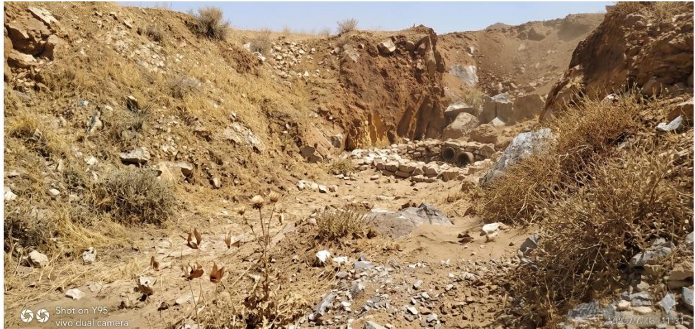
Fig: 16 Garland drains with clarifiers
