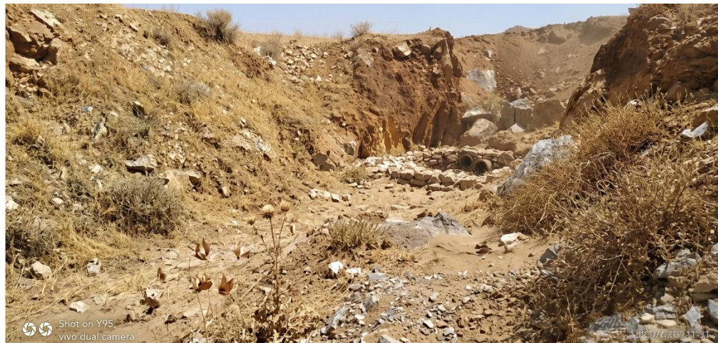
Fig: 9 Garland drains with clarifiers
